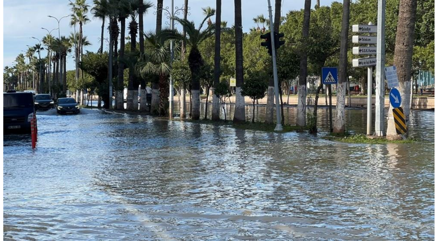
Subsidence of Iskenderun City
